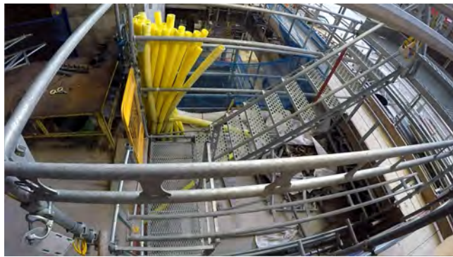
Figure 32. Exit to North and South Cores via external temporary scaffold dogleg stairs on the ground level of 22 BG.
