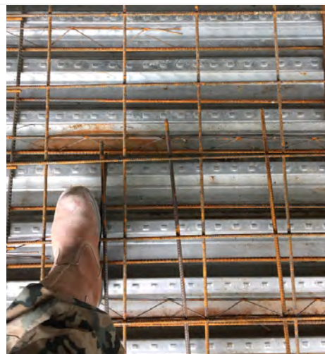
(b) Metal decking with rebar.
