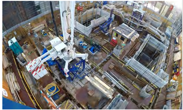
View from camera (23) in slipform.
