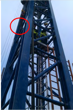
Camera (23) being setup in slipform.
