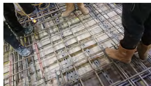
(f) Decking with rebar.
