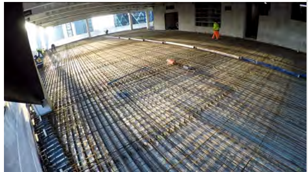
View from camera (7) on Level 7 on floor.
