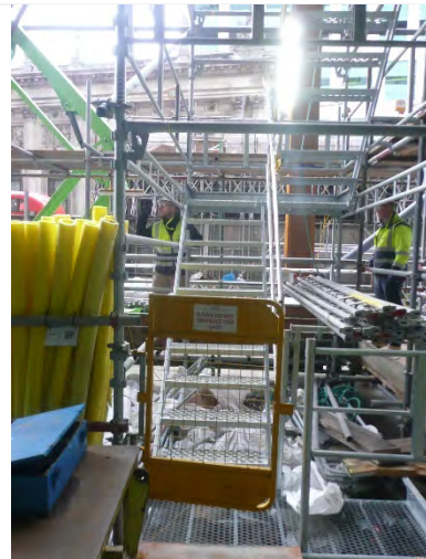
Figure 32. Exit to North and South Cores via external temporary scaffold dogleg stairs on the ground level of 22 BG.
