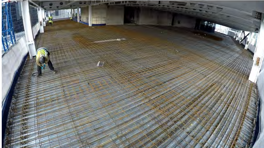
Figure 50. Worker installing rebar.
