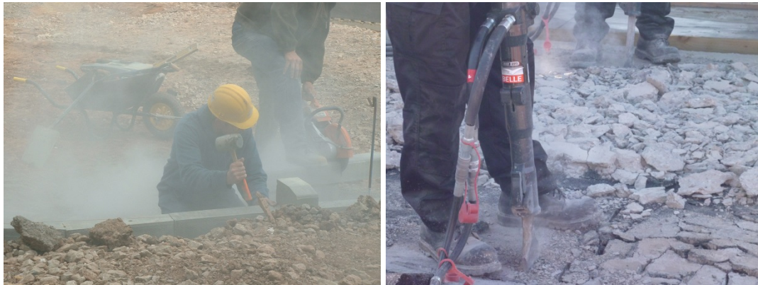
Figure 19 Typical construction and demolition activities, releasing concrete dust
