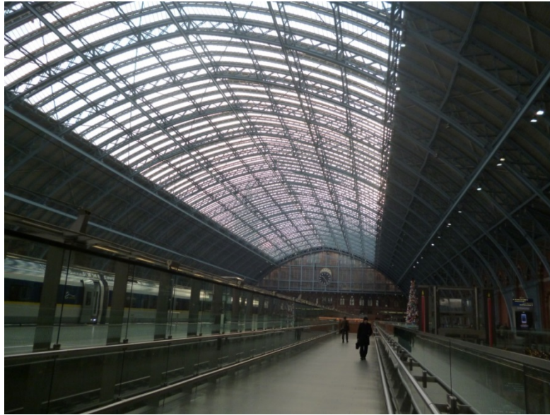
Figure 8 The roof of St Pancras station in London reportedly has self-cleaning glass
