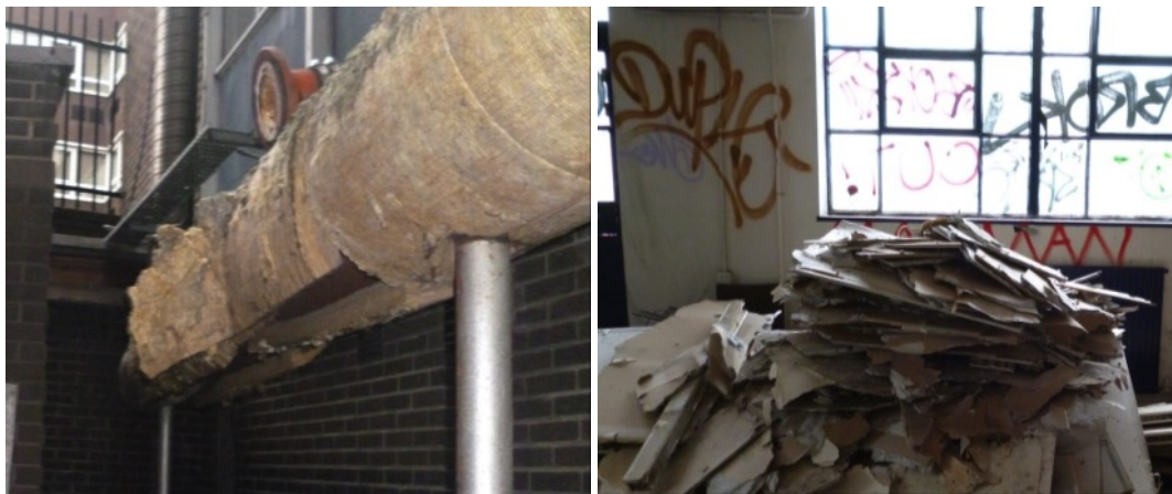
Figure 26 Insulation materials and plasterboard removal during demolition
