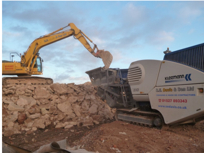
Figure 21 A concrete crusher which will break down waste concrete, bricks etc.
