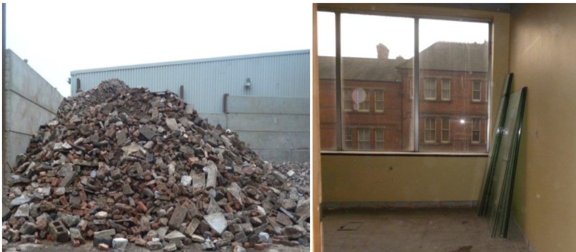
Figure 24 Small fragments of glass will be mixed in with waste aggregate. Larger pieces may be recycled into new float glass
