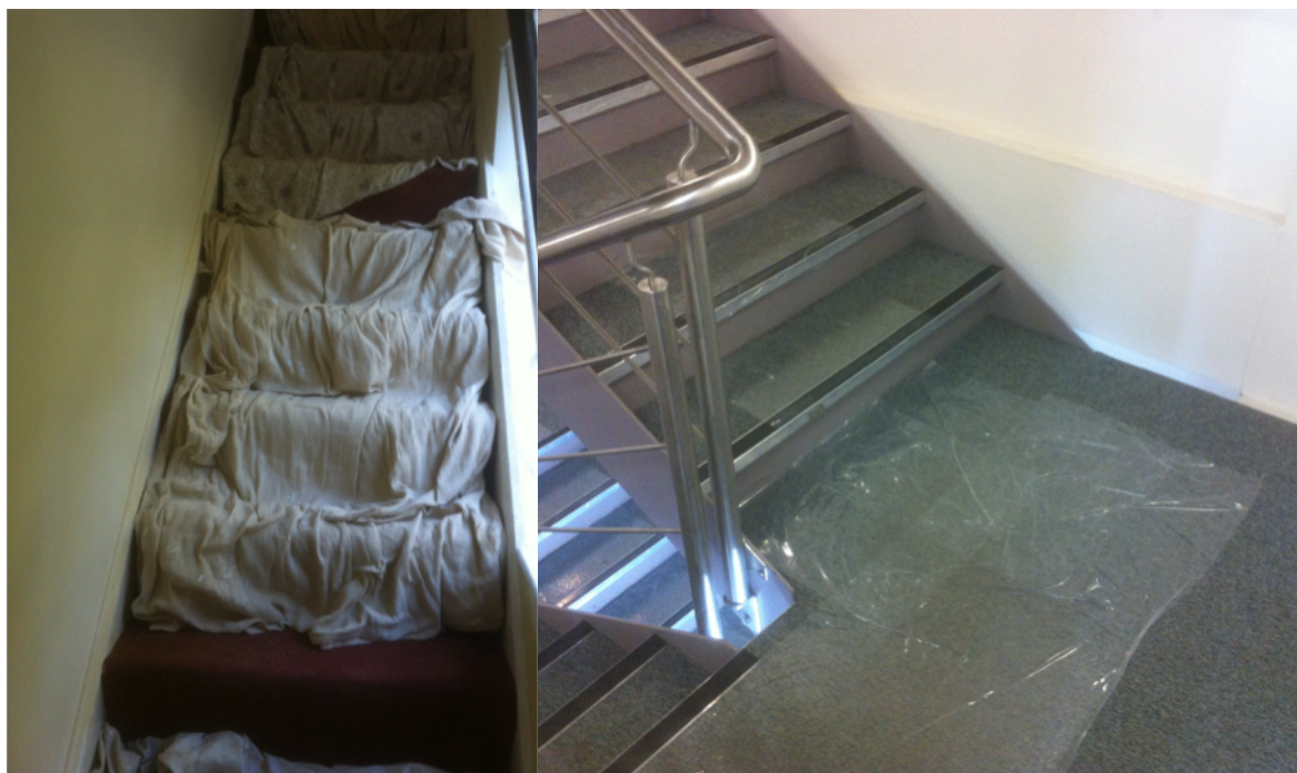
Photo 4.4: Trip hazard from dust sheet used by micro organisation to protect homeowner’s carpet with more appropriate protection used by a larger firm on a major commercial project (Photo Gibb).
