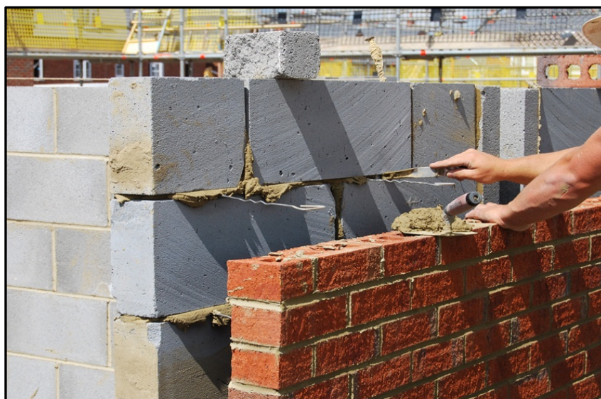
Figure 3.12 a bricklayer described feeling through the trowel for the “right” consistency of mortar, and developing physical proficiency working with this material
