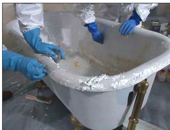
Workers use a methylene-based stripper to remove paint from a bathtub prior to refinishing.
