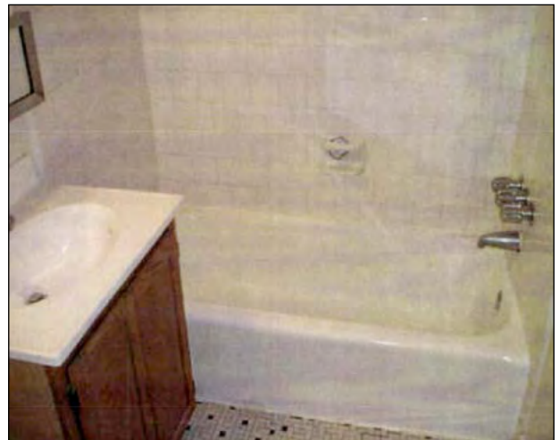
Photo courtesy of Maryland Occupational Safety and Health
