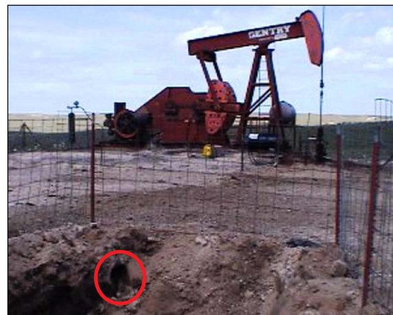
Cut end of pipe in trench.
