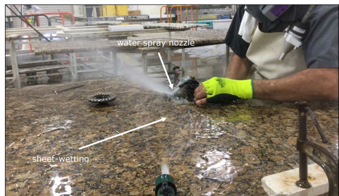
A worker uses an angle grinder with a diamond grinding cup wheel to finish a stone countertop. Combining “sheet-wetting” with a water spray nozzle helps reduce RCS exposure during grinding. Photo by NIOSH.
