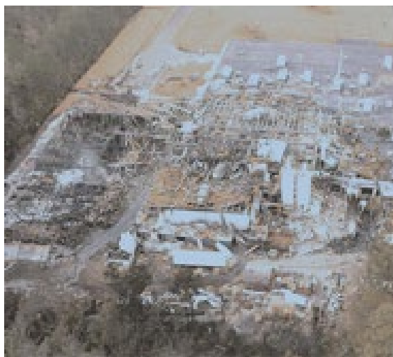
A pharmaceutical plant after a dust explosion.
