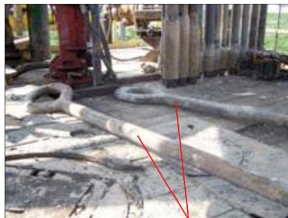
18-foot bales dropped to the rig floor.
