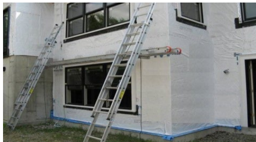
Ladder Jack Scaffold
