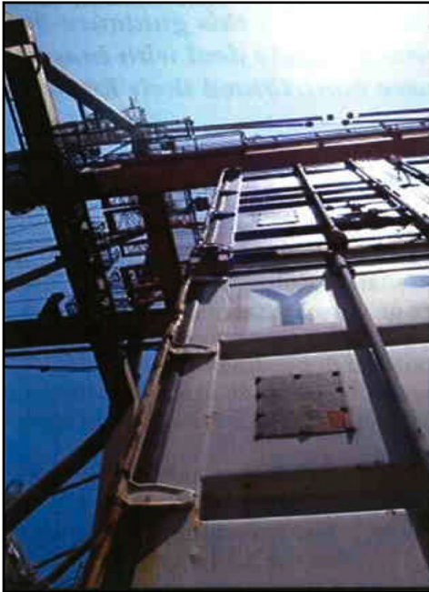
Foreman must direct the crane operator's movement.
