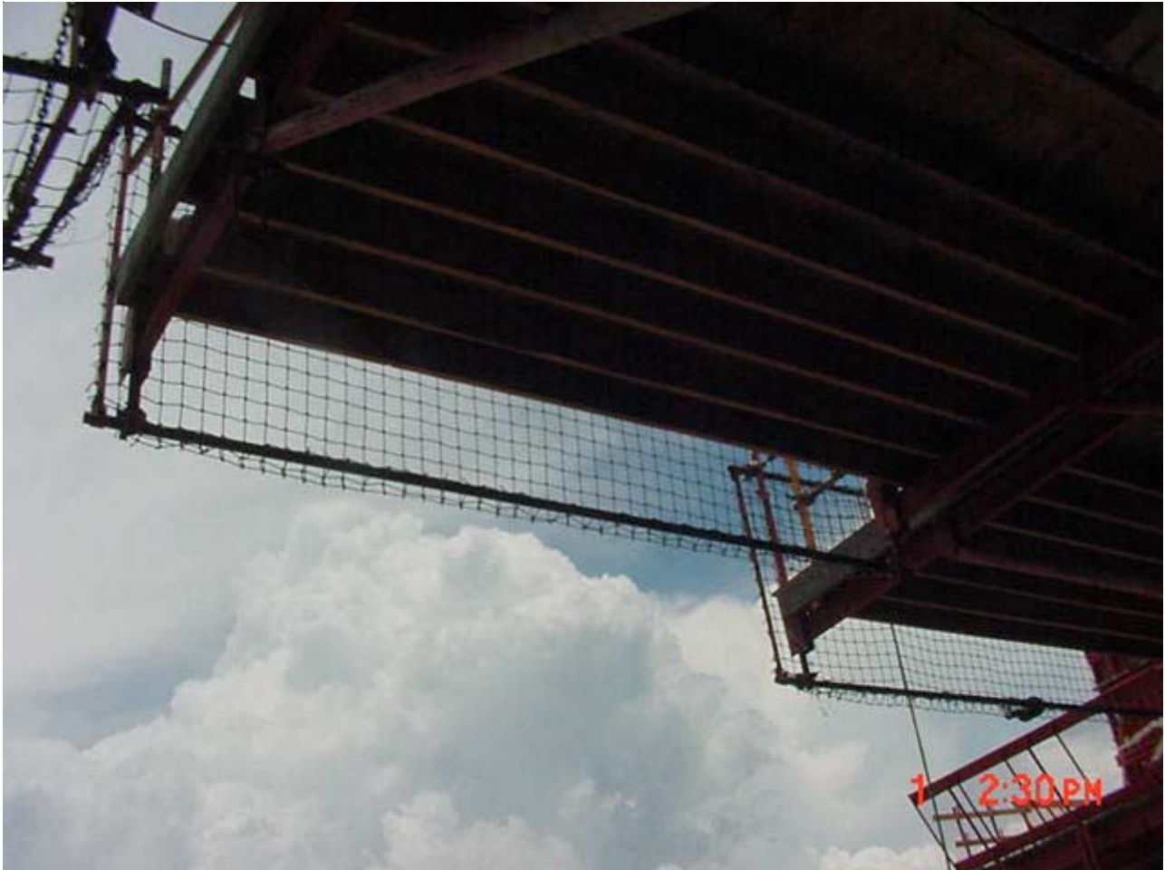
Underside of Stripping Platform showing mesh guarding.
