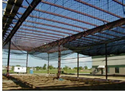
Safety nets used in construction sites.
