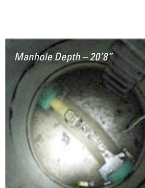
Figure 1: Photo of manhole
