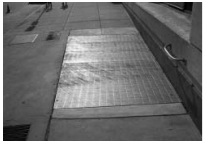
Figure 4. New Grate System
