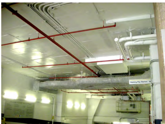
Figure 8.1. A fire sprinkler system.
