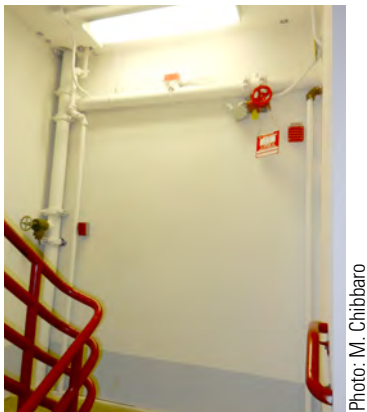
Figure 9.19. A standpipe isolation valve on a feed main (entering horizontally from the upper right) leading to a vertical standpipe riser (on the left). The valve is located within the stair enclosure to protect both the valve and the firefighters who may need to access it.
