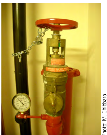
Figure 9.6. An FHC equipped with a pressure-regulating device.
