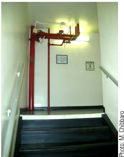
Figure 8.6. A sprinkler zone control valve in a stair enclosure.
