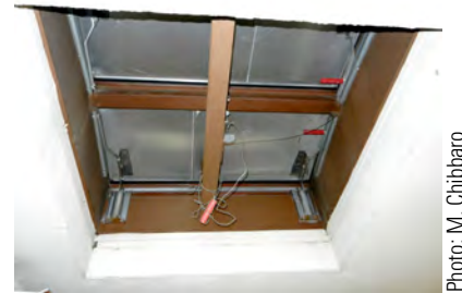
Figure 12.15. A smoke vent at the top of a stair.
