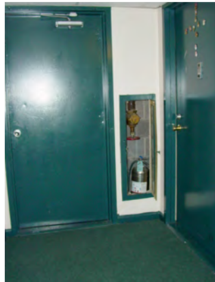
Figure 9.15. A FHC on the corridor side of a stair door (on the left).
