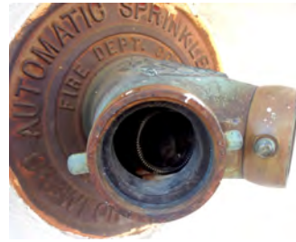
Figure 13.13. An FDC with a glass bottle jammed into one inlet.
