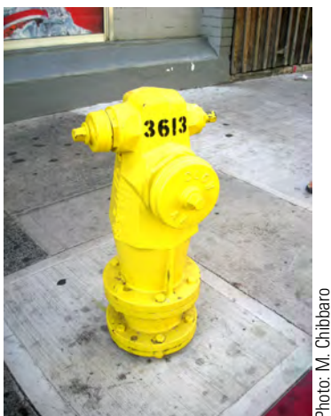
Figure 4.6. A wet barrel fire hydrant. The operating nut for the small hose outlet is on the right. The operating nut for the large outlet is on the rear of the hydrant.
