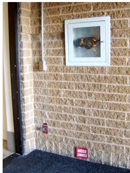
Figure 9.9. A remote FHC in a cabinet in a corridor. The sign near the floor is intended to help locate the cabinet in light smoke conditions. Note that the hose outlet is angled to facilitate connection of hose.
