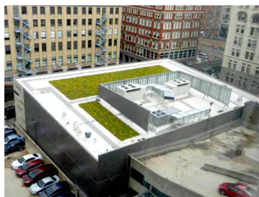
Figure 7.15. A vegetative roof system with paths that could be used for access and ventilation.
