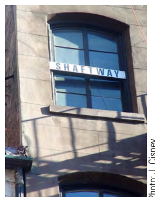
Figure 7.10. Exterior shaftway marking.
