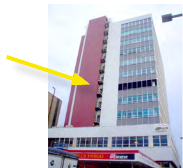
Figure 9.18. An exterior view of open air vestibules (arrow) between the stair and the interior of a building.
