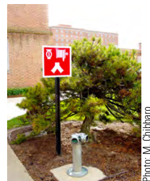
Figure 10.14. An FDC sign with the NFPA 170 symbols for both sprinkler and standpipe systems.
