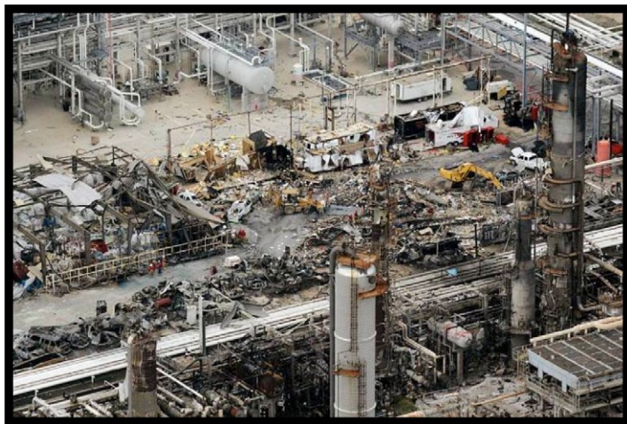
An explosion at a refinery site killed 15 and injured nearly 200; an idling diesel pickup truck was the most likely ignition point.
