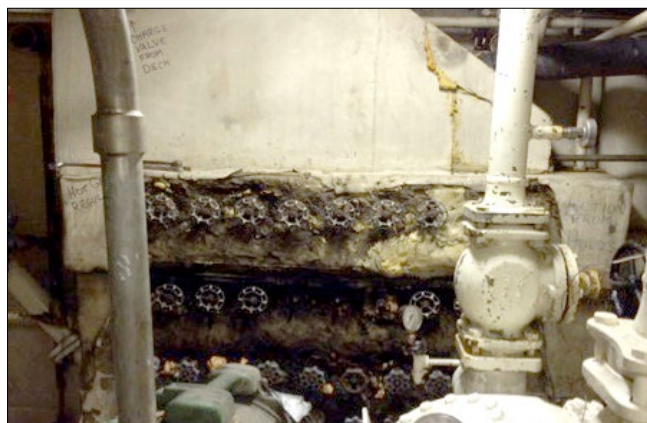
Examples of refrigeration systems aboard vessels.
